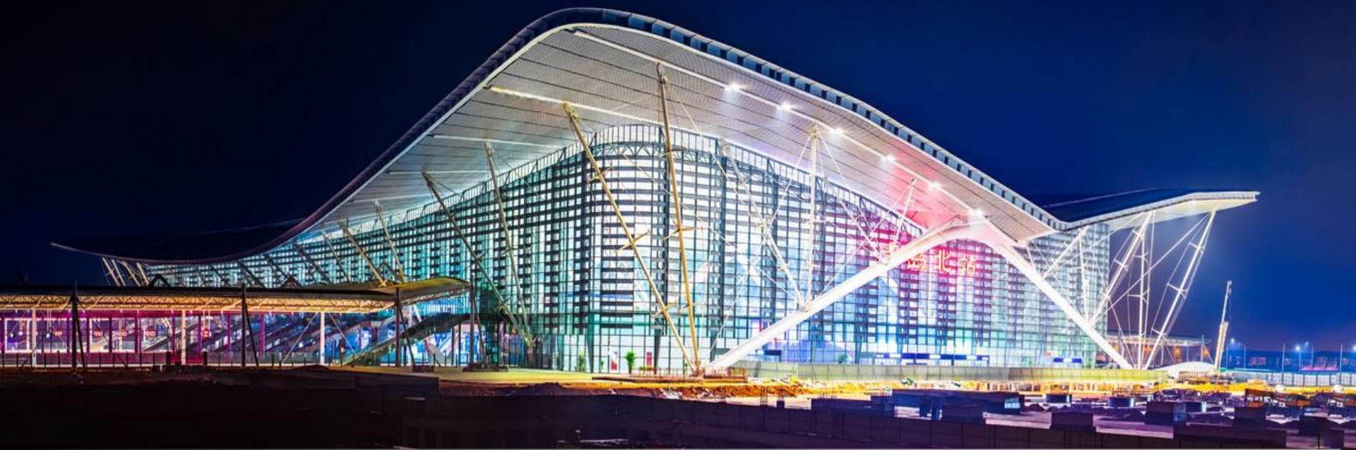
Shandong-Qingdao North Coach Station Podium Building
